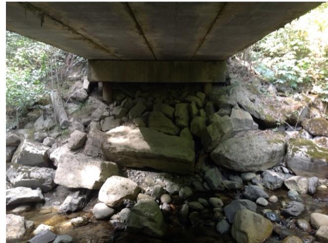
Right Bank Abutment when facing downstream
