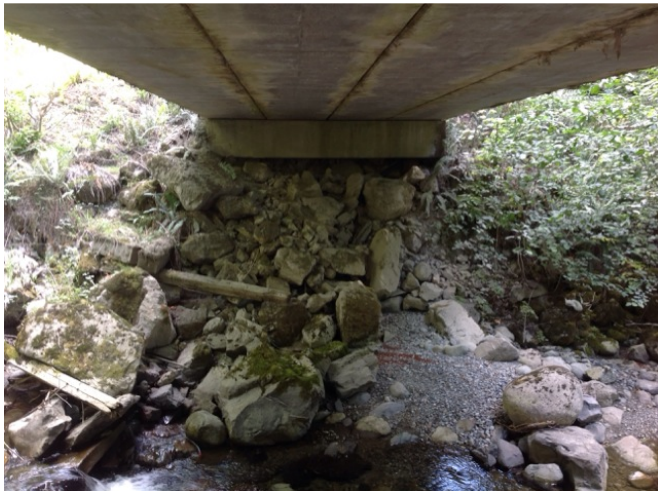
Left Bank Abutment when facing downstream
